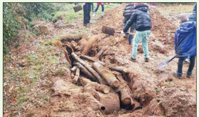
The hibernaculum under construction
