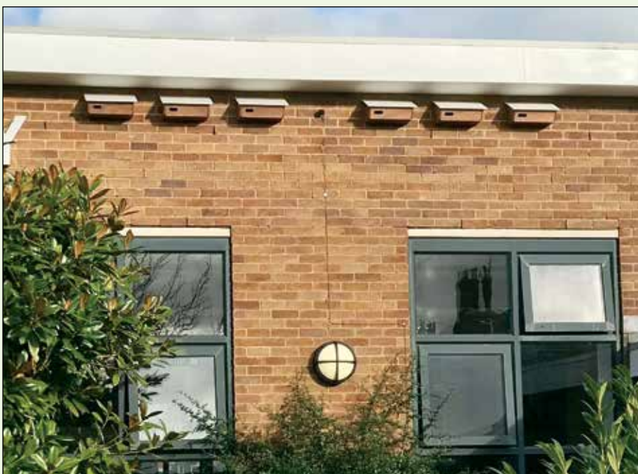
Swift boxes installed at Felixstowe library
