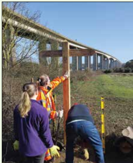
Volunteers installing new signposts
