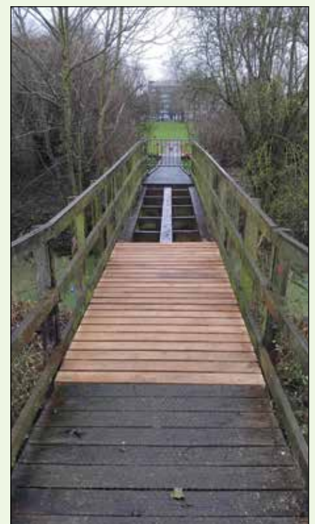
New oak deck on bridge at Alderman canal.
