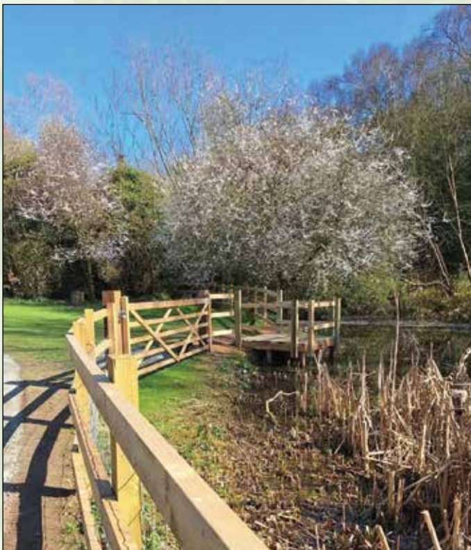
The new fencing around the pond and dipping platform
