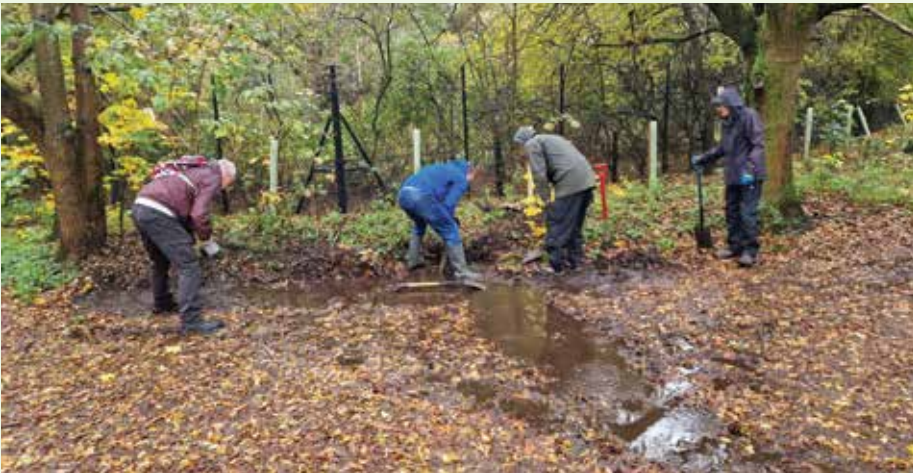
Urgent work clearing the drain
