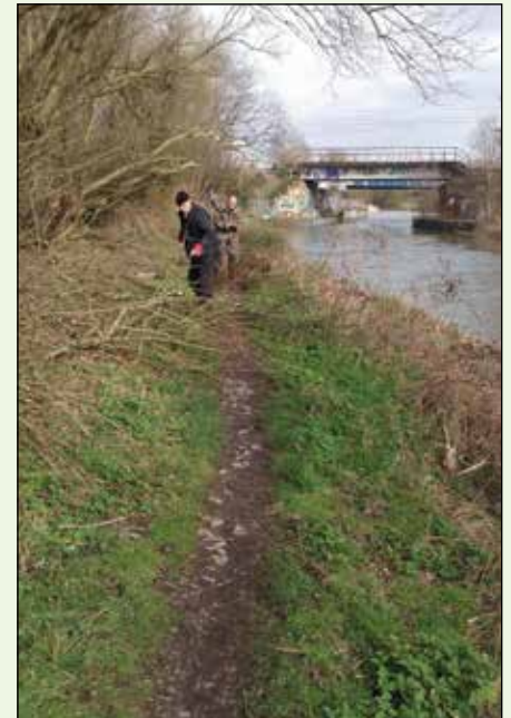
Vegetation clearing before widening the path
