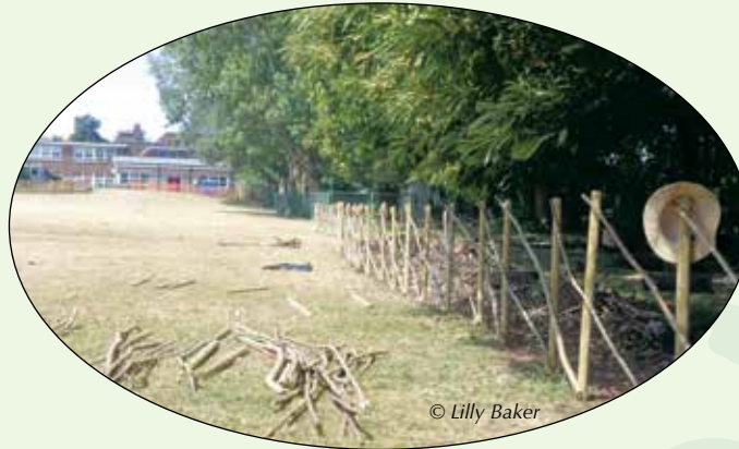
Hazel fence under construction at Hillside School
