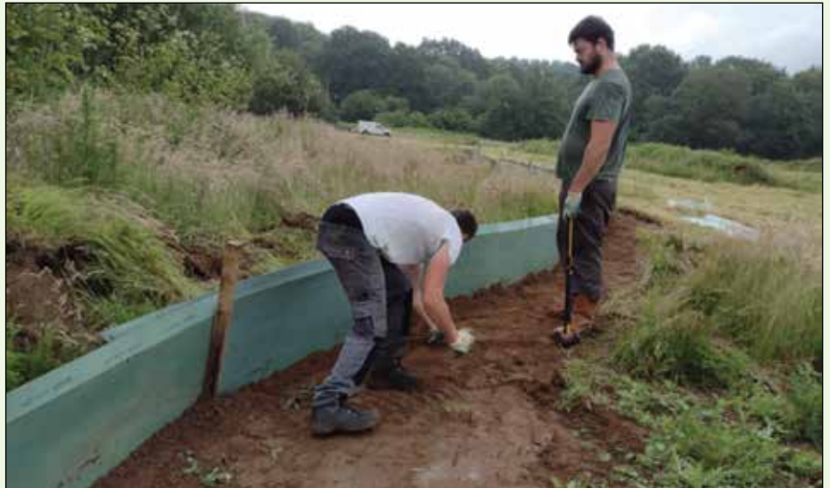
Partitioning off sections of the fields using reptile fence panels
