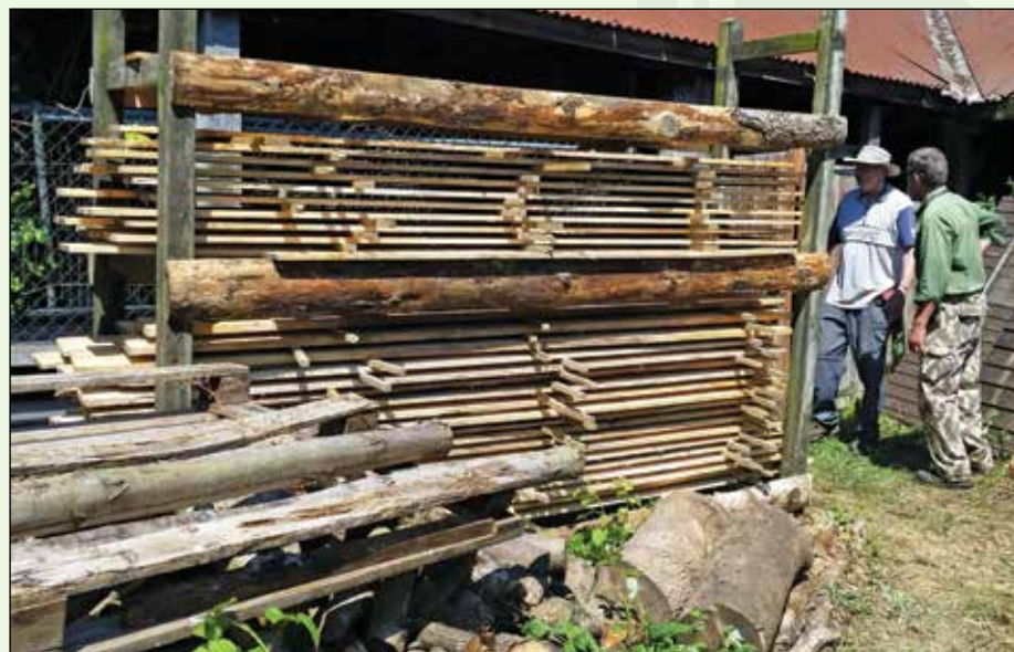
Completion of a project by our Friday Barn work party to construct racking to allow timber planks, produced by the Greenways mobile saw mill, to air-dry before being used to make wildlife homes for birds, bugs, bats and hedgehogs.
