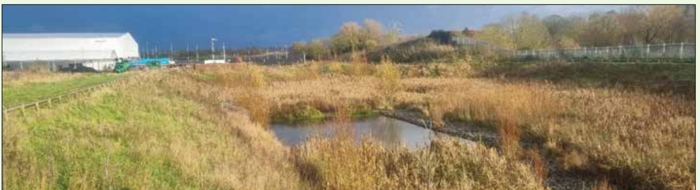
Sustainable Urban Drainage system close to the river, with Amazon warehouse in the background.
