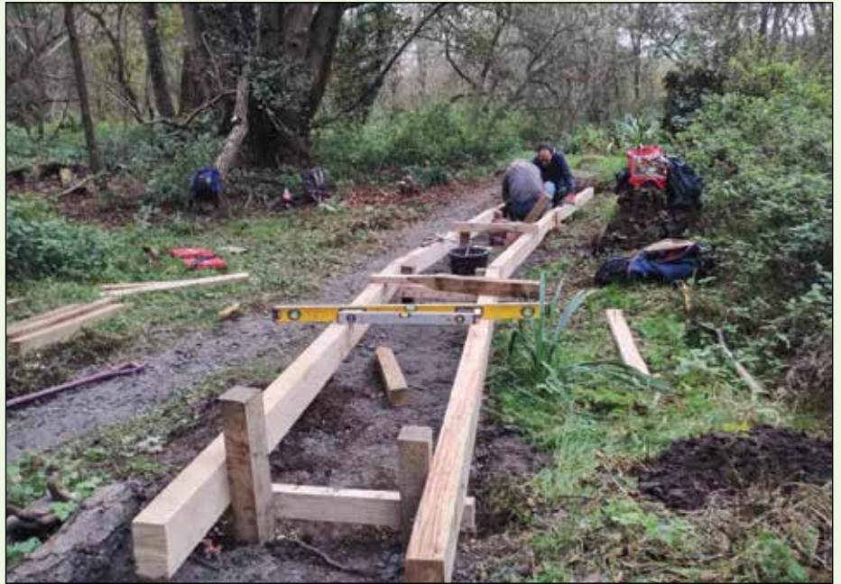
Boardwalk under construction using local oak
