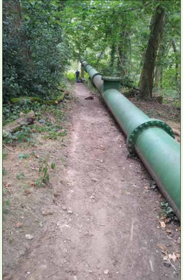
The Ashground Plantation 'Poo pipe'
